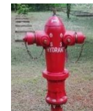
Gambar 10. Hidran pillar
