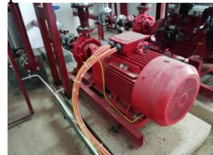
Gambar 7. Electric main pump
