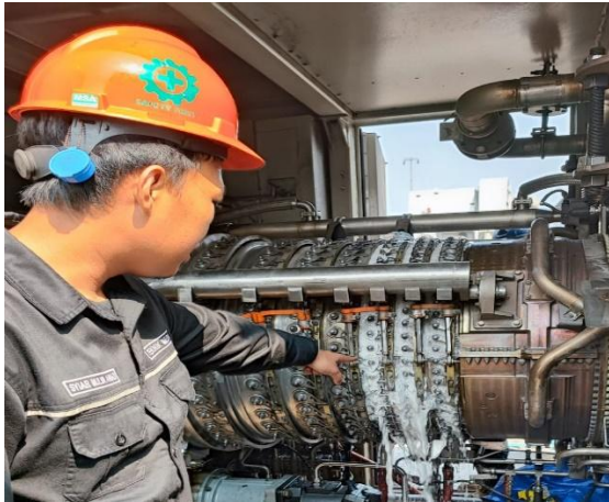
Gambar 3 Pelaksanaan Water Wash Compressor
