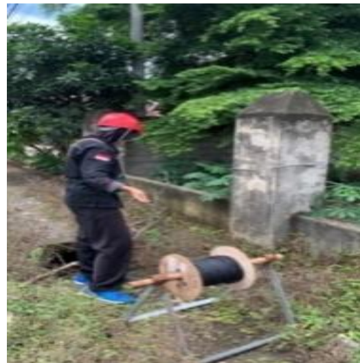
Gambar 3 Penarikan kabel fiber drop core
