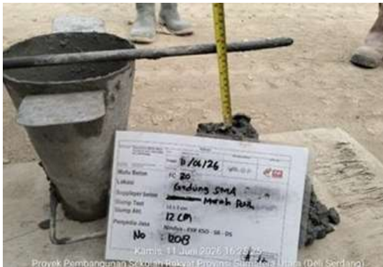
Gambar 8. Slump Test Ramp Gedung SMA
